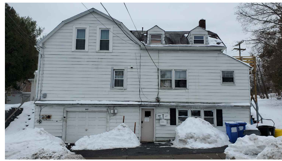
PHOTO EXISTING EAST MAIN STREET ELEVATION
