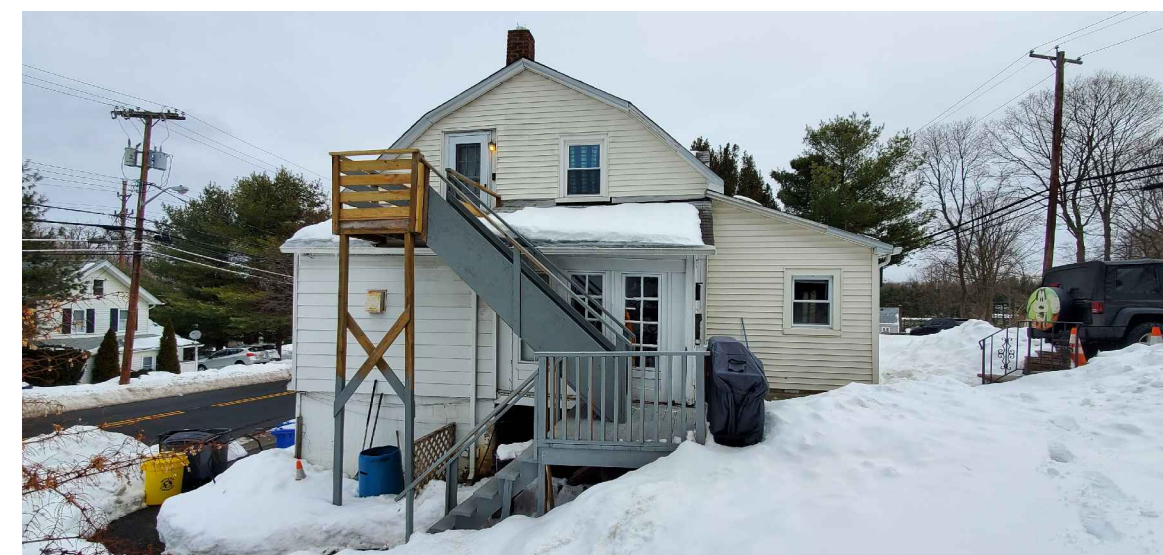
PHOTO EXISTING LEFT SIDE ELEVATION
